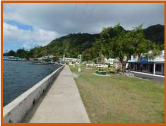
Rebuild of the seawall
