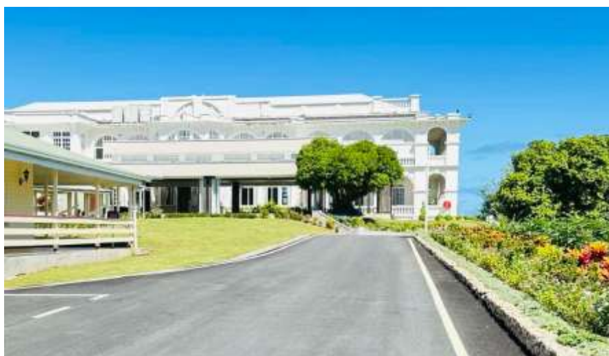
Now – after major restoration works.
