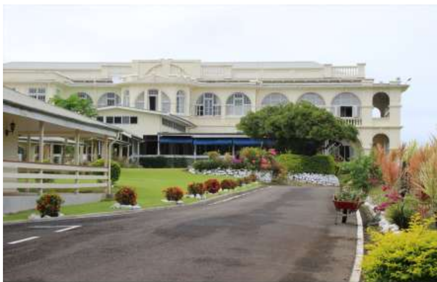
Then – before refurbishment works
