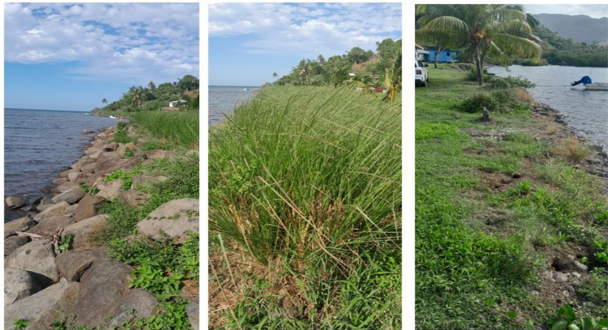
Illustrations 5.14 – 5.16: Seawall with boulders and planted vetiver grass with incomplete village seawall.
