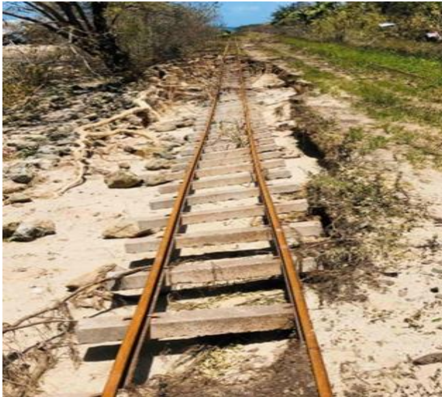
Damage caused by TC Yasa to Rail Tracks in Daku Sector
