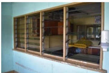
Figure 3: Missing louvre blades
