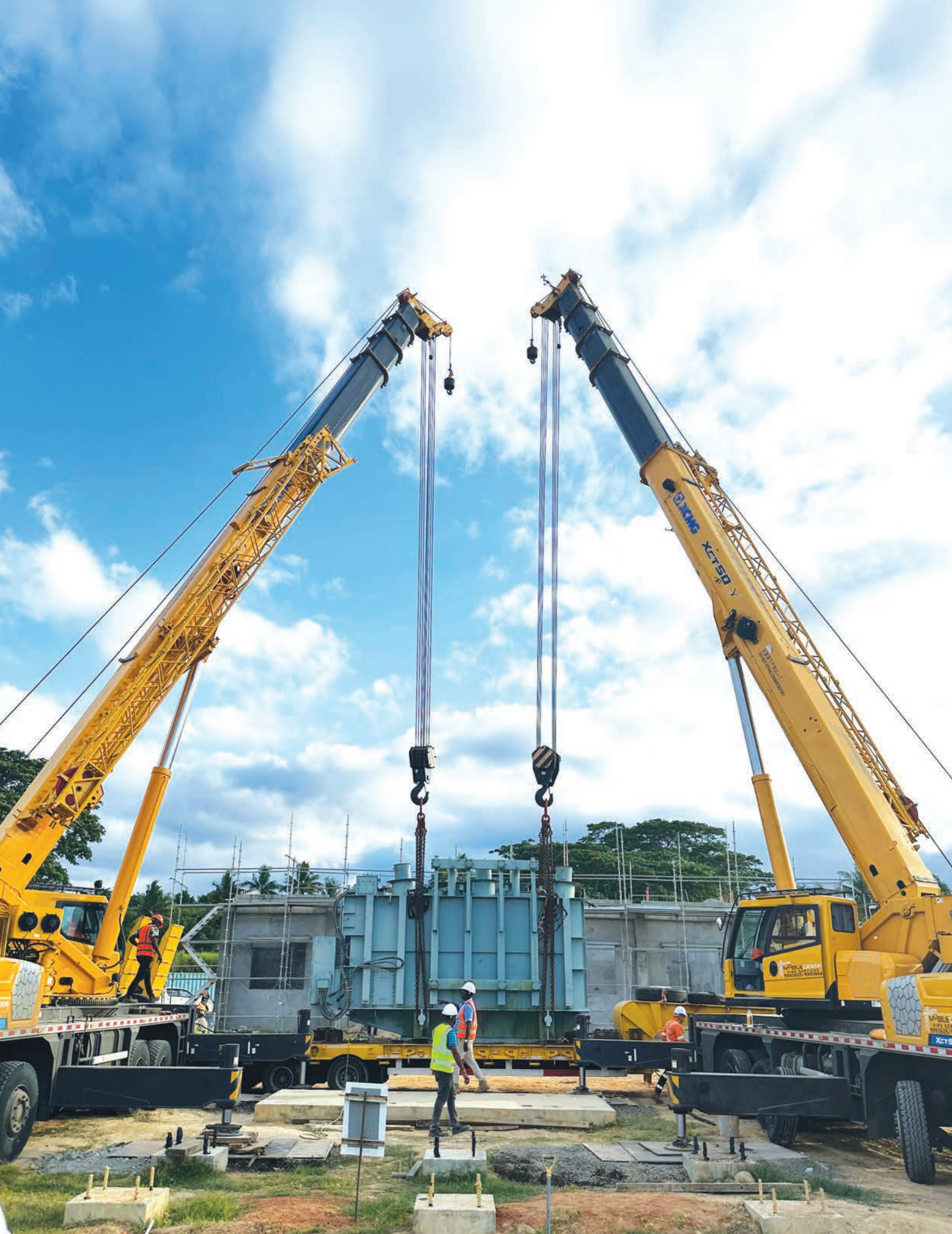
Installation of 132/33Kv Transformer on Pad at Koronubu for Virara to Koronubu, Ba 132kV Transmission Line Project.
