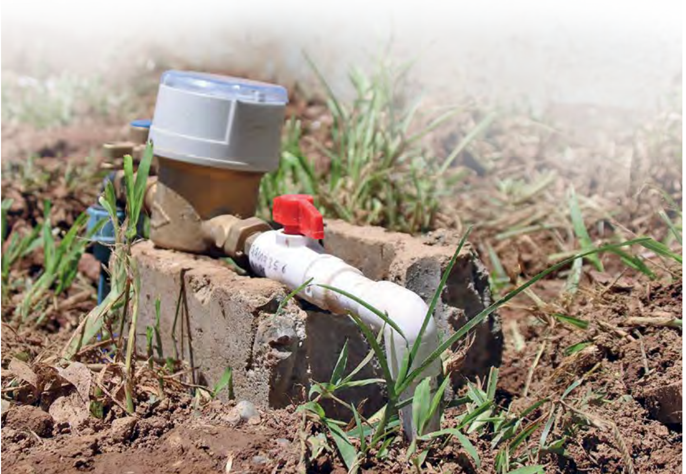
A newly installed water meter.
