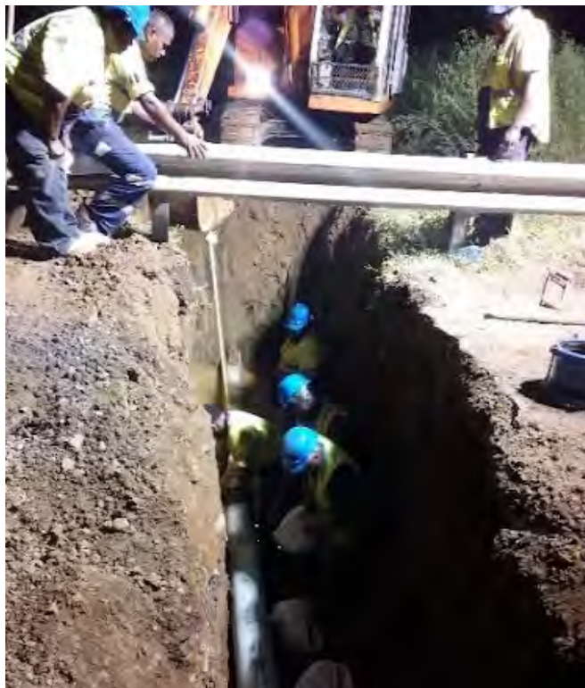
Re-alignment of 200mm PVC pipe between Duilomaloma and Corbett Avenue junction.
