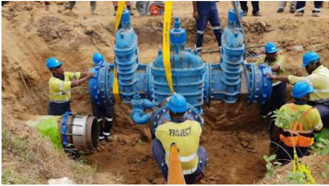
Commissioning of the new DN600 pipeline and system balancing
