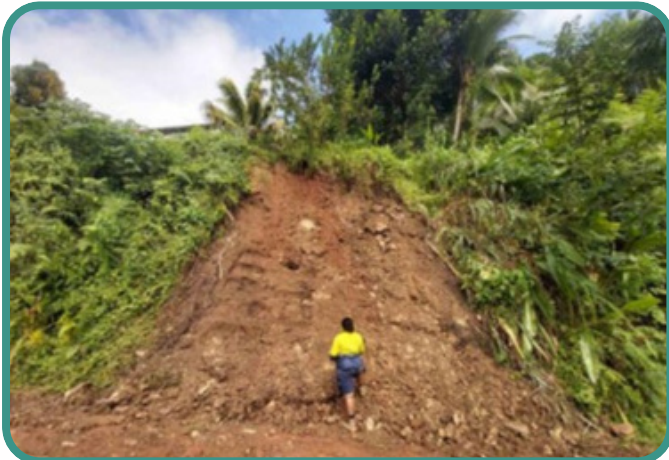
Minor Slip identified on a road cut near Wainadiro village, Serua (left) Shallow slump located inland in the Waidradra area, roughly 1km north from the Main Queens Road (right)
