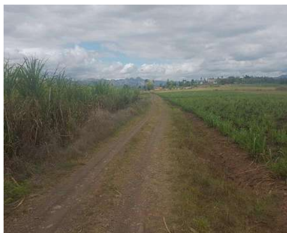
Road repaired under the CAR Project
