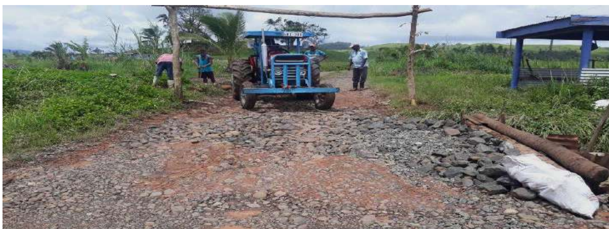
Growers of Waiqele Sector Repairing Road after TC Ana
