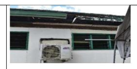
Figure 84: Metal pipe attached to ceiling may fall down
