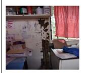
Figure 76, 77, 78 & 79: Water leaking resulted in deteriorated condition of walls around door, powerpoint (circled), underneath shelves and next to sink.
