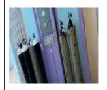
Figure 32: Oxygen cylinder stored on passage way which can fall down
