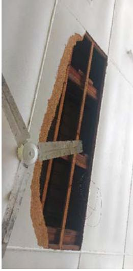
Damaged ceiling in classrooms, there are also instances sighted where the ceiling is hanging loose and can fall on someone
