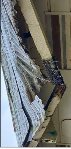
Rusted and damaged roofing iron and old gutterings
