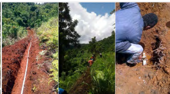
Laying of water pipes and installation of air valves at Natadradave Village, Tailevu.
