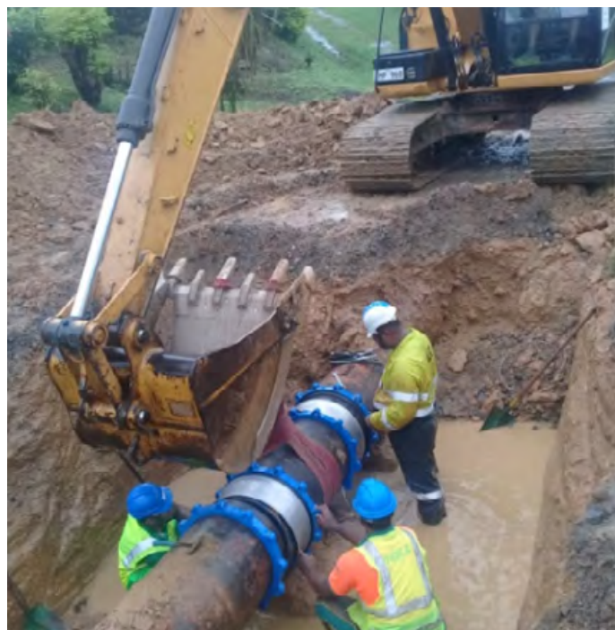
Rehabilitation & Recommissioning of the old DN 600 Trunk Mains from Vaturu to Nagado WT
