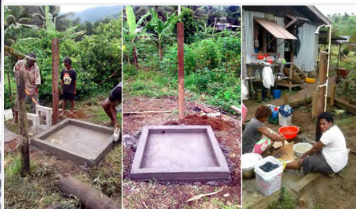
Construction of concrete slabs and standpipes at Natadradave village Tailevu
