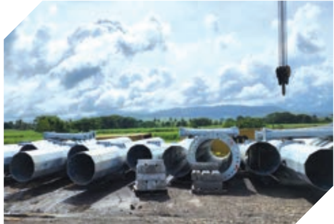
EFL received steel monopoles and lattice towers for the new 132kV Virara to Koronubu Network project.
