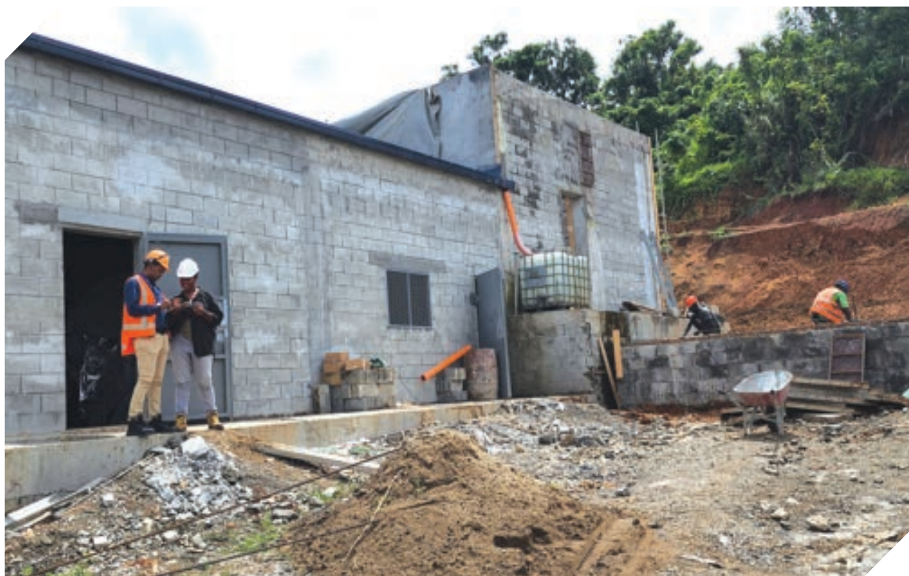
Waitolu 33kV/11kV zone substation under construction and expected to be completed in 2023. This substation will be part of the Viria water reticulation project.
