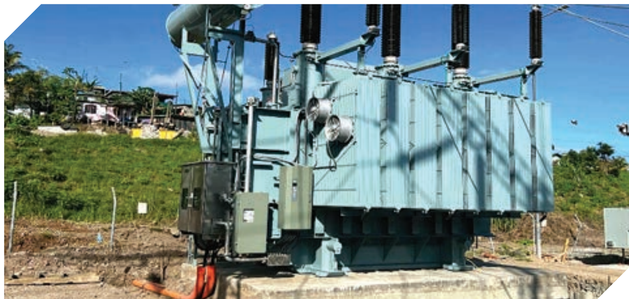
Installation of the new 132kV/33kV T2A Power Transformer at Cunningham Road Switch Yard.
