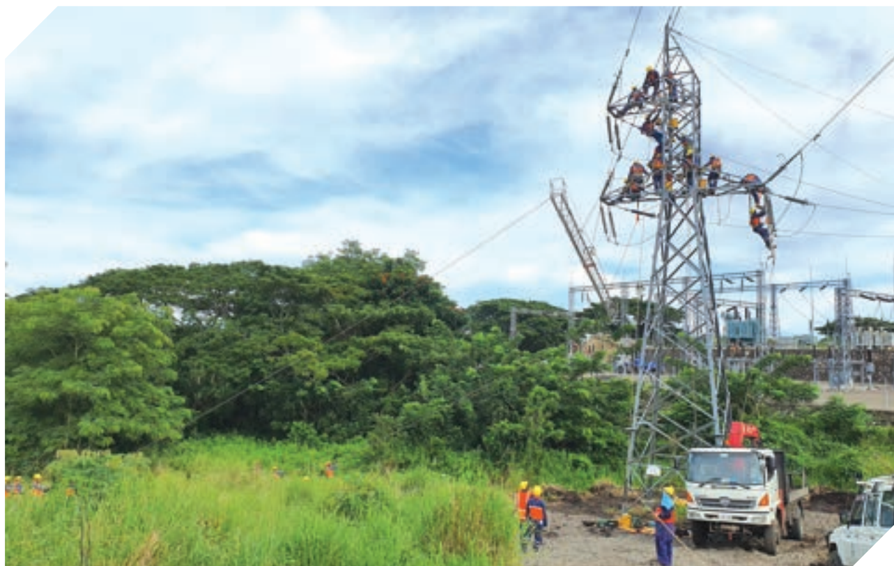
EFL Transmission Team carrying out maintenance on the 132kV Transmission Tower near Vuda Substation.
