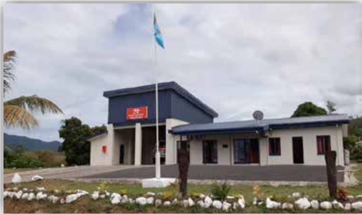
Newly constructed Rakiraki Fire Station.
