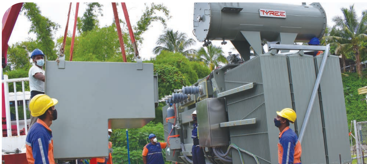
Assembly of the new 33kV/11kV,6.6kV transformers at the Suva Zone substation being carried out to meet the growing energy demand in the Central Division.
