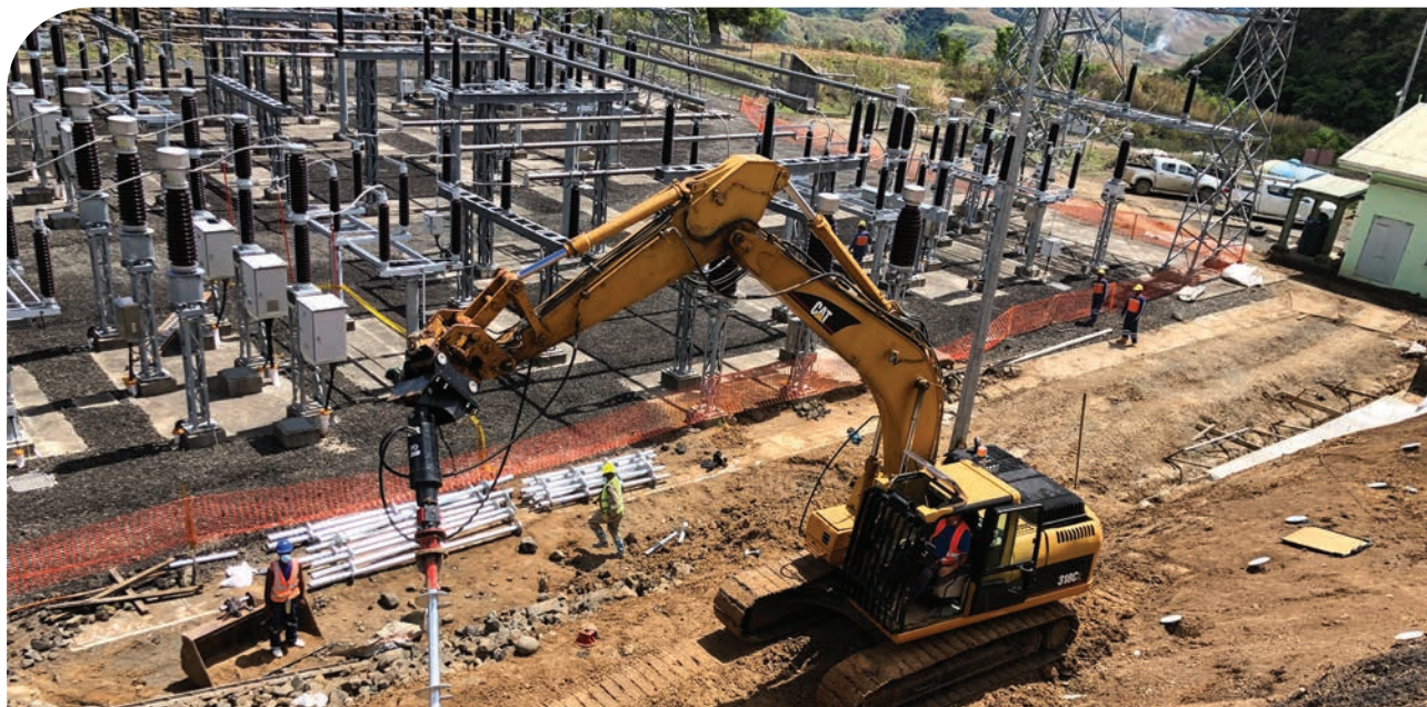
Land soil nailing works to stabilise landslide at the Nadarivatu switchyard
