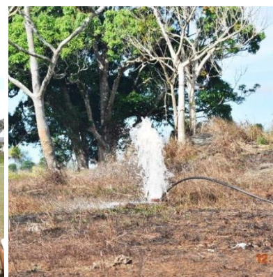
Figure 23: Cleaning of existing borehole using high capacity method
