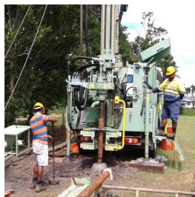
Figure 22: Groundwater exploration drilling underway using mud rotary method
