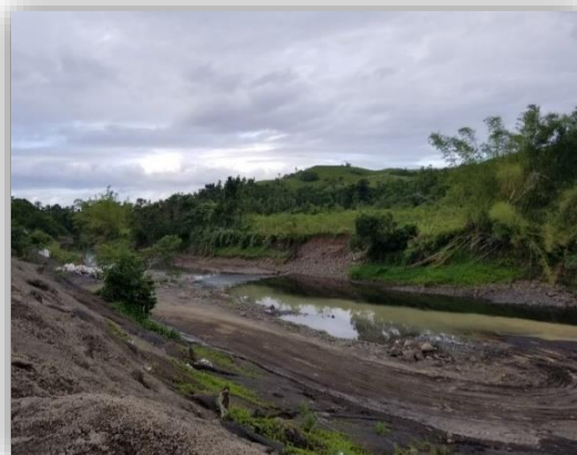
Figure 5.12 & 5.13: Excavator tracks towards the river with muddy sediments being discharged in the river
