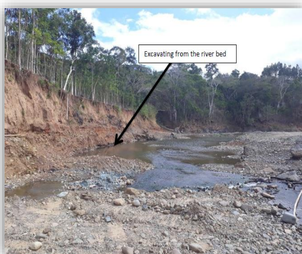
Figure 4.17: Bank collapse into the diverted water way
