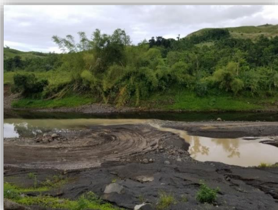
Figure 5.12 & 5.13: Excavator tracks towards the river with muddy sediments being discharged in the river
