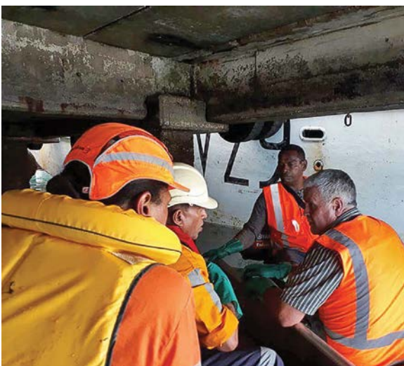
▲ Port of Mua-i-Walu 1 repair and inspection.
