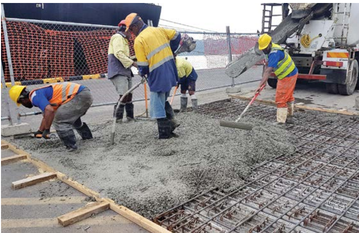
▲ Lautoka Local Wharf deck rehabilitation.
