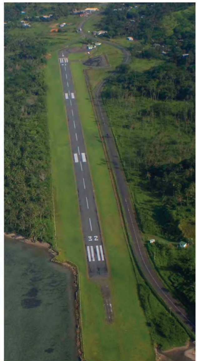
An aerial view of the Savusavu runway.
