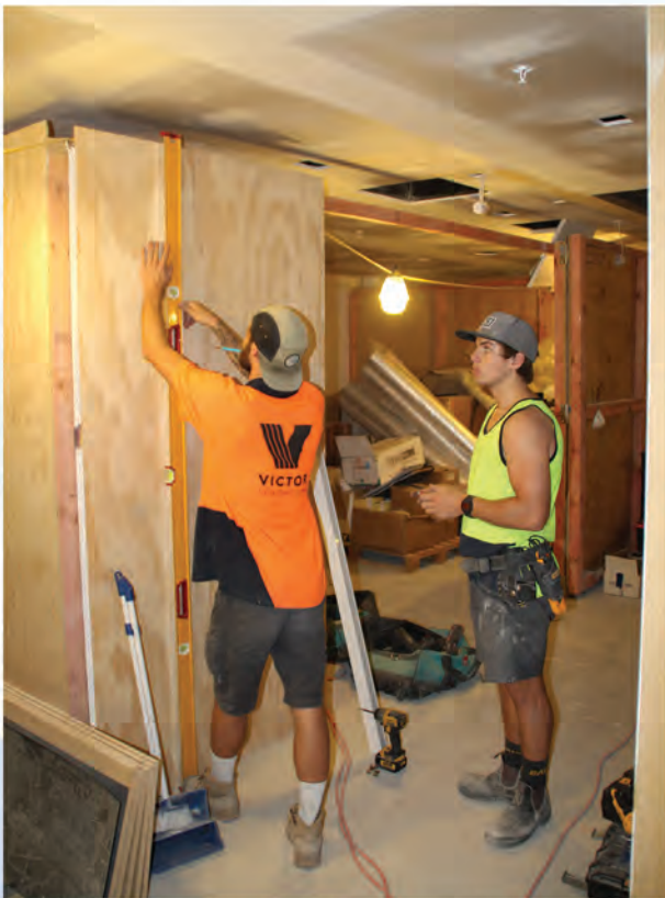
During the construction of the new Air NZ VIP Lounge.
