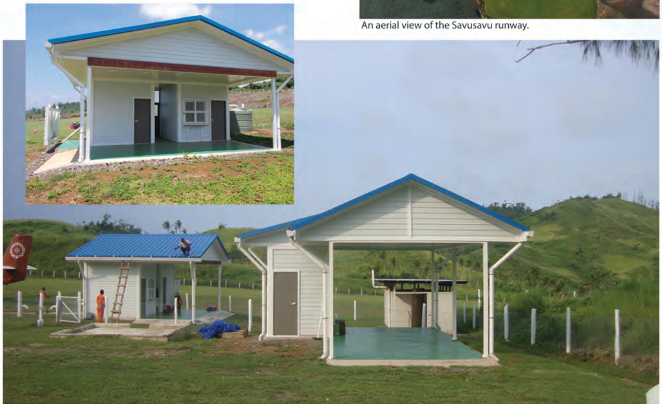
Our Koro and Vanua Balavu terminals were rebuilt after being significantly damaged by TC Winston.
