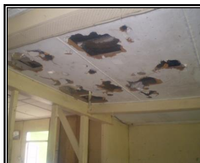
Deteriorating ceiling
