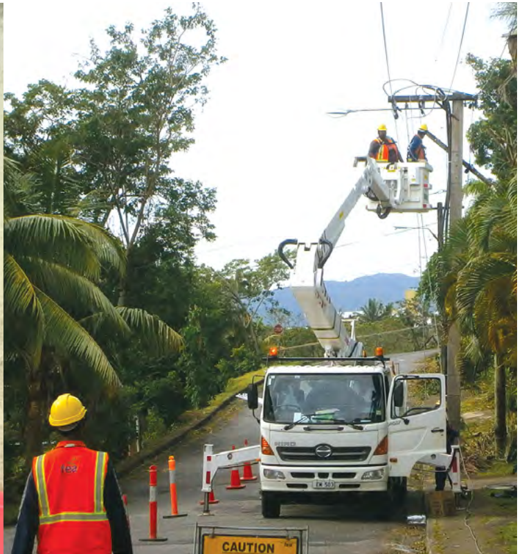
The FEA liveline team maintaining the overhead transmission line to ensure reliability and security of power supply to customers.
