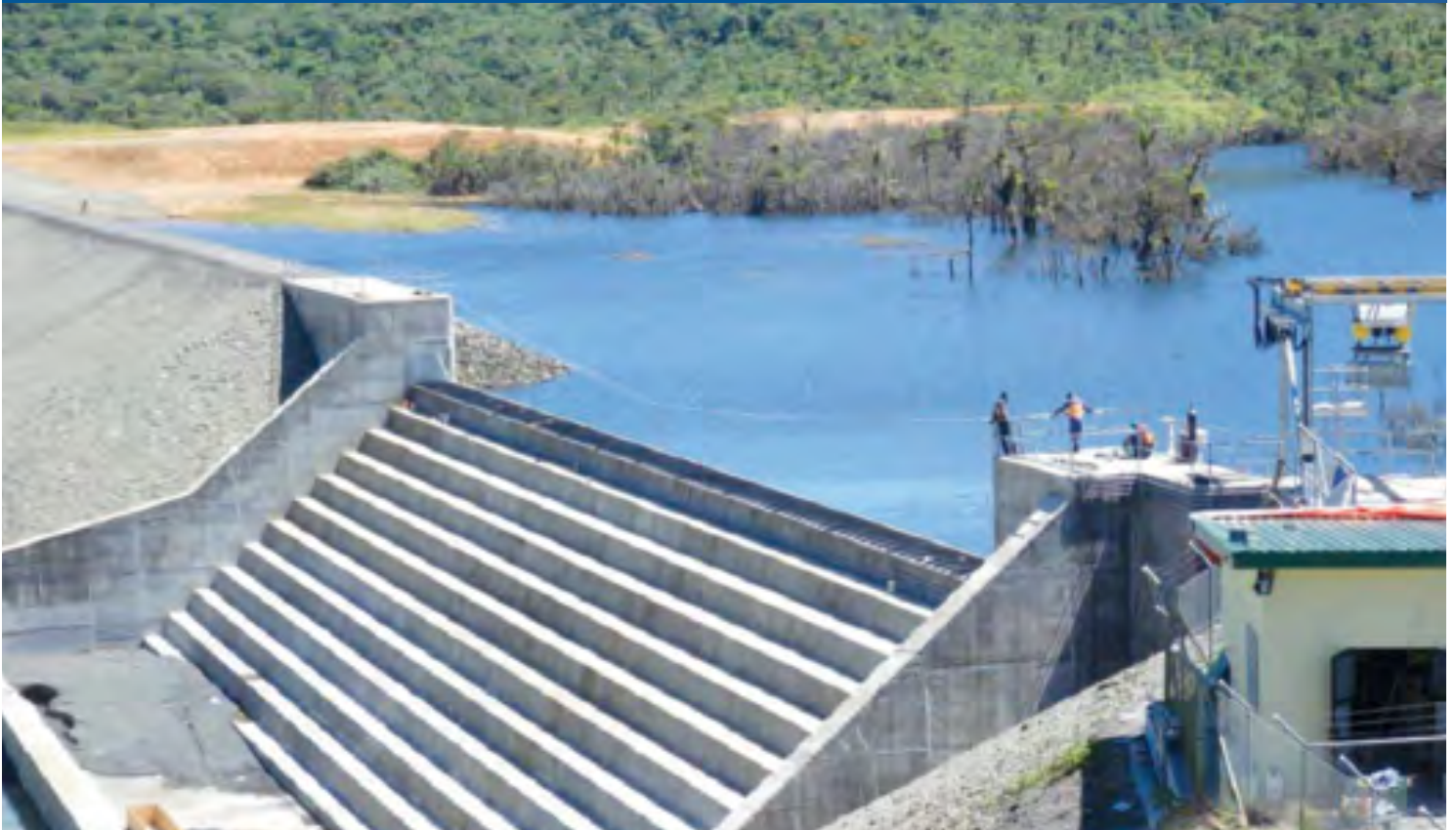
FEA commissioned the Wainisavulevu Weir Raising Project (WWRP) on 3rd of November 2015. The raising of the weir by an additional 8 metres will increase the energy output from the two existing hydros namely Wainikasou and Monasavu Hydro-electric Schemes and is expected to achieve a fuel savings of around $4M per annum.
