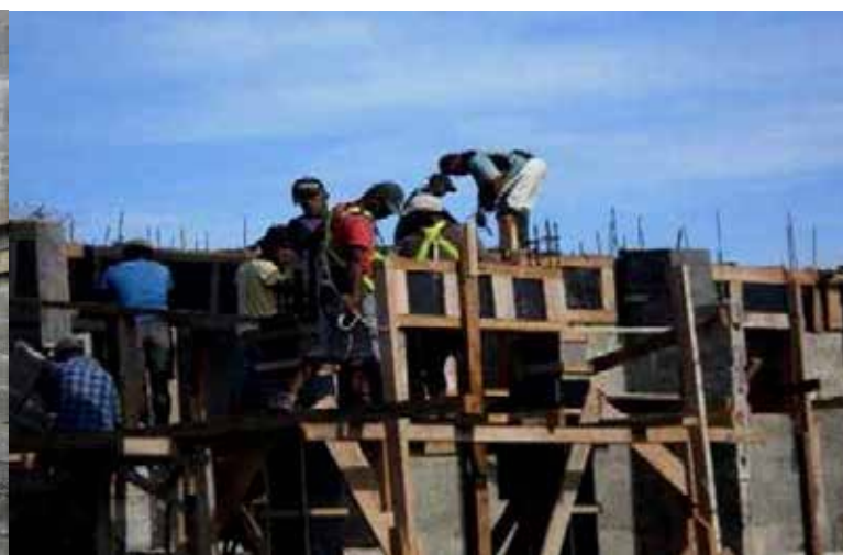
Figure 3: Naqere Housing Project
