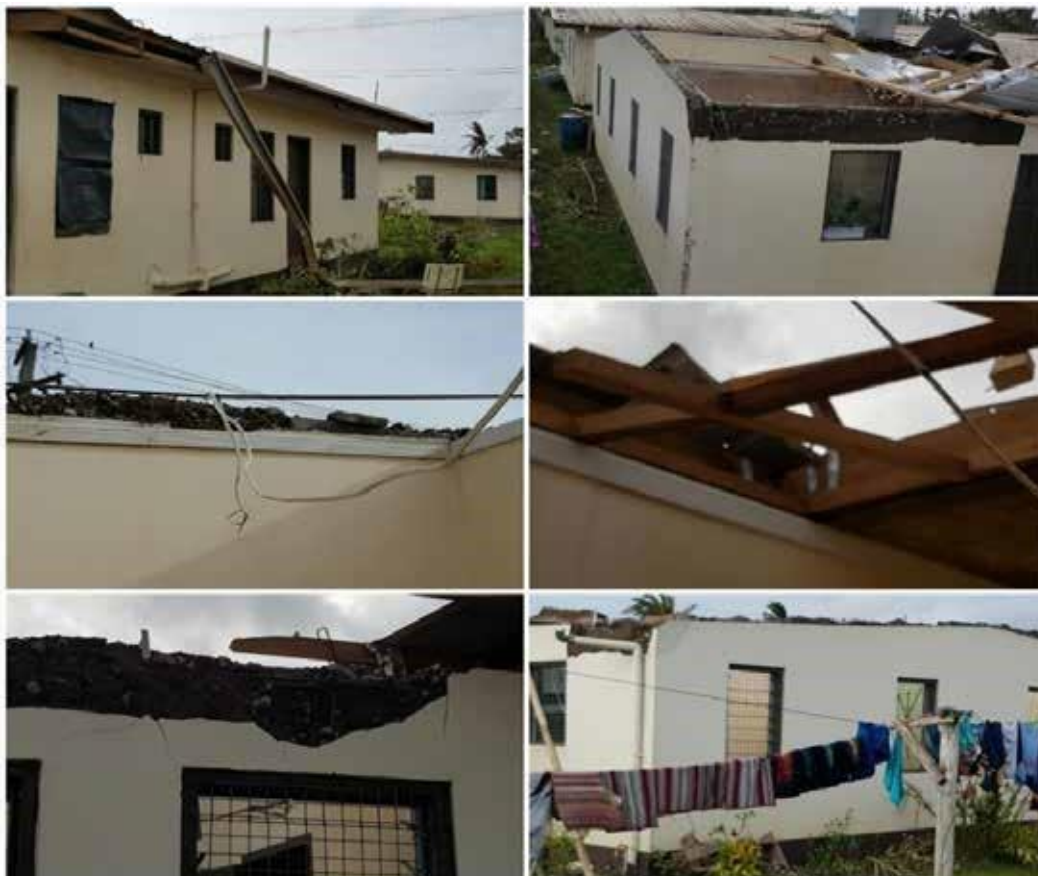
Figure 4: Pictures showing the damages sustained by 2 x 4 flat buildings at Lovu, HART Community, Lautoka.
