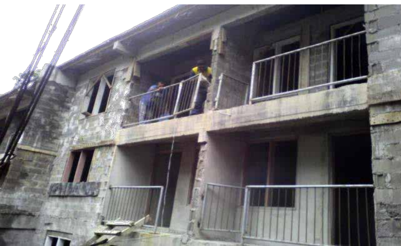
Figure 2: Kalabu Housing Project
