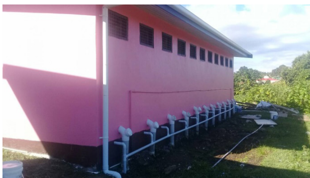
Figure 9: Renovation to Suva Methodist Primary School, Suva
