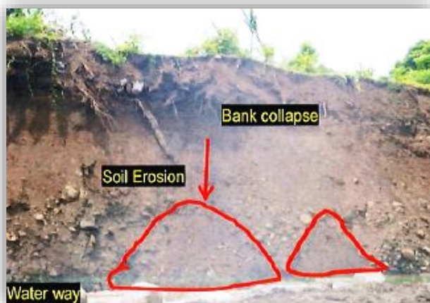
Figure 4.15: Bank collapse into the diverted water way
