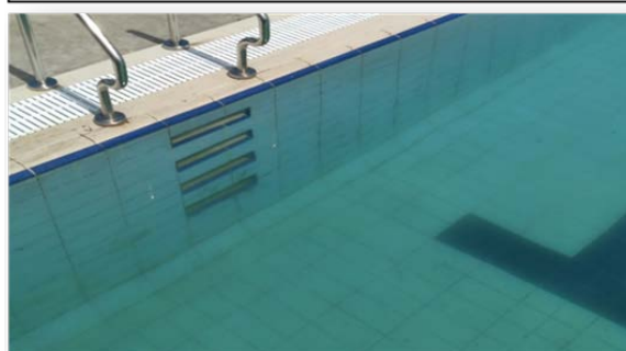
Pool Steps (Incomplete) and Drain - Training Pool
