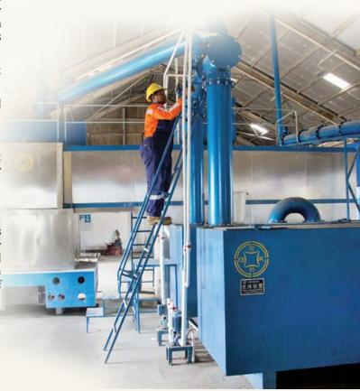
Conforming to FPCL's Green Port Initiative and Company's commitment towards the reduction of emissions, the new electric powered incinerator was installed and commissioned by the Engineering Team with the engagement of an Engineering Consultant of the overseas supplier at a cost of FJ\$630K.
