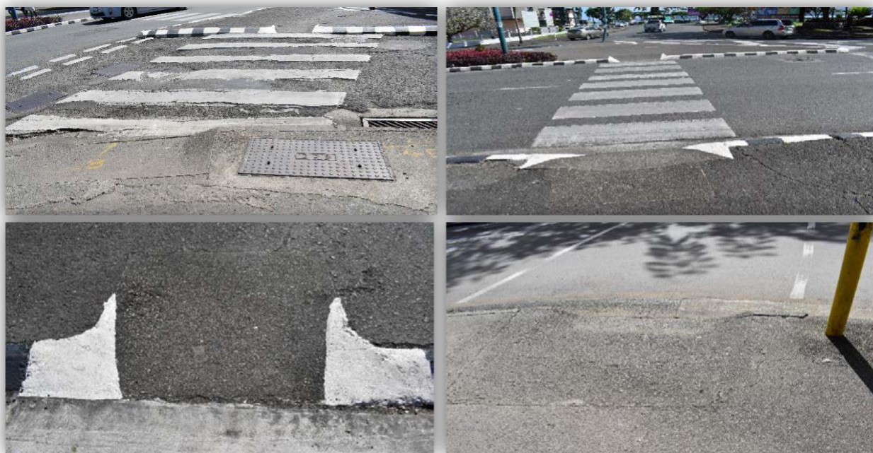
Figure 5.11: Inconsistent measurement of curb ram
