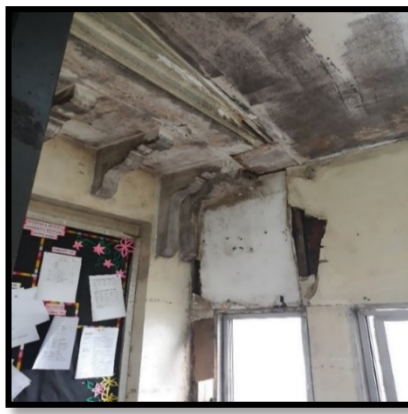
Figure 30: Damaged ceiling in dietician's room
