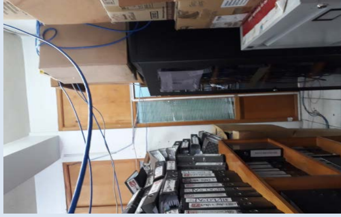
Exposed wires running through the passages (walking area)
