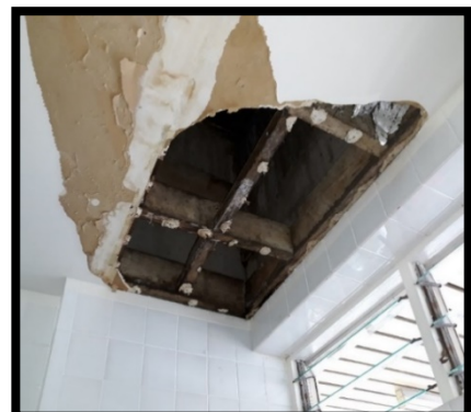
Figure 12: Damaged ceiling for staff bathroom at Maternity Unit
