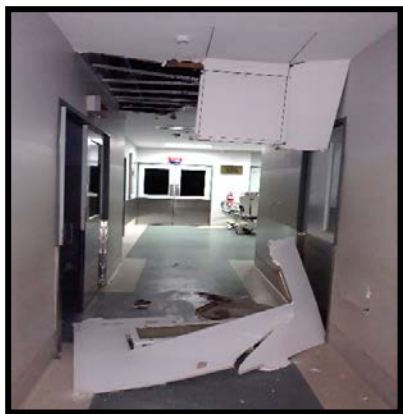
Figure 32: Collapsed ceiling at the new operating theatre
