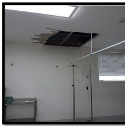
Figure 31: Open ceiling at the new operating theatre recovery room
