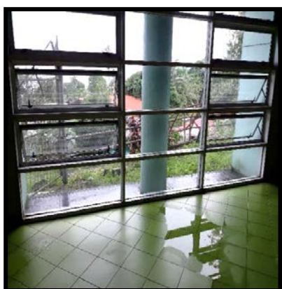
Figure 29: Water leaking into Dental Department
