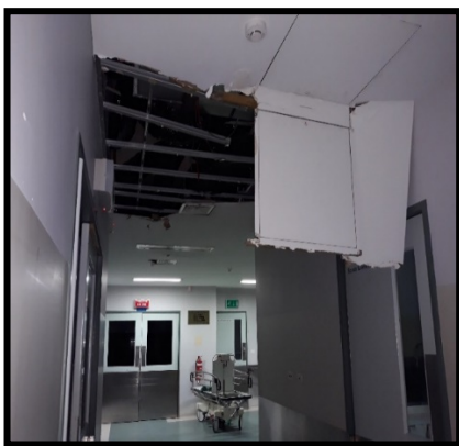
Figure 33: Collapsed ceiling at the new operating theater
