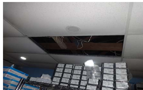
Figure 6: Missing ceiling from pharmacy. Medicine are exposed to heat from the roof.
