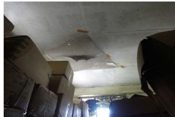
Figure 3: Leaking roofs - plastic attached to ceiling to collect water
