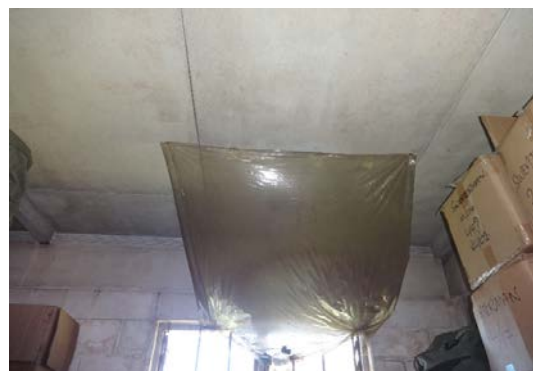
Figure 4: Plastic attached to ceiling to collect water
