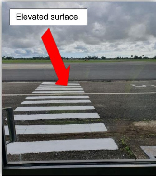
Figure 5.93: Evenly surfaced boarding area with elevated surface on runway
