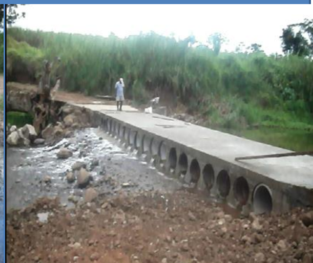
Figure 2: Qalitu cane access crossing (Irish crossing) after CAR programme.
