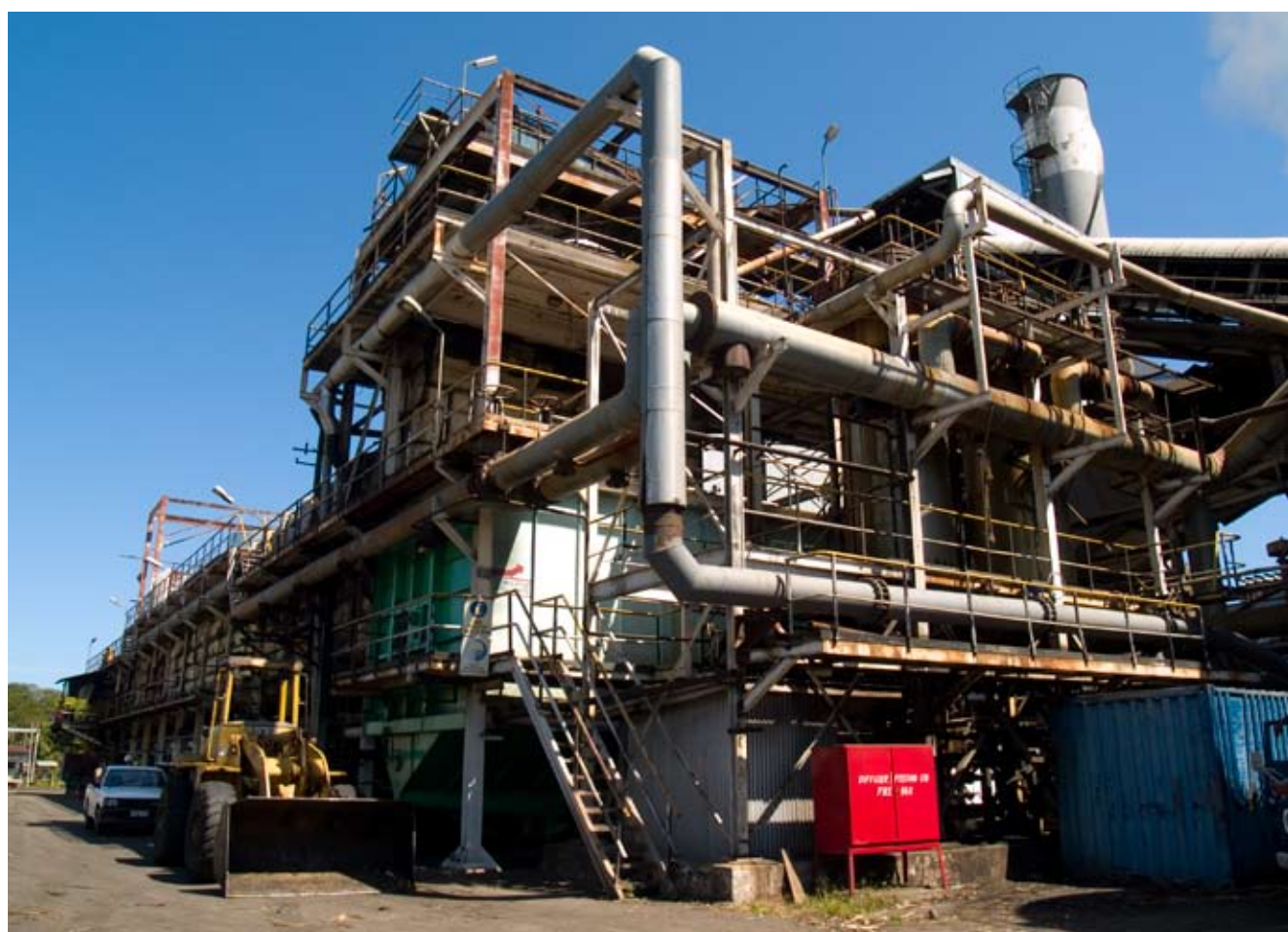
The Extractor Plant separates the juice from the sugarcane.
