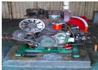
Figure 3 Diesel Electricity Generator - Duel Fuel Kits
