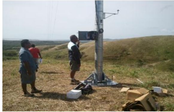
Figure 4: Wind Tower installation in western Viti Levu
