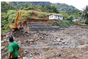
Re-excavation to divert river to its normal course at Suweni village
