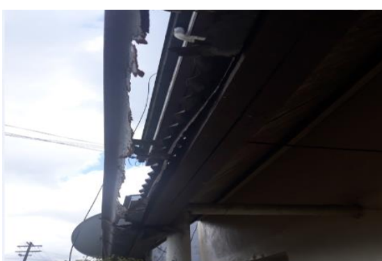
Figure 20.20: Old guttering needs replacement
