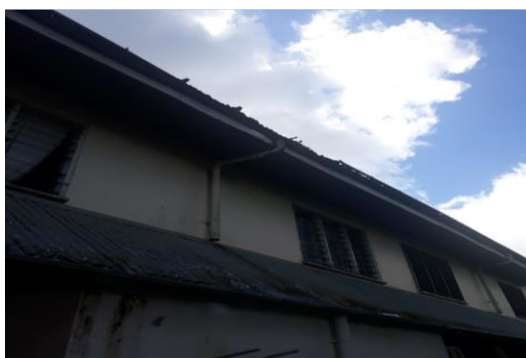
Figure 20.17: Roof/guttering needs replacement
