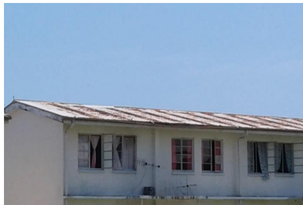
Figure 20.24: Rusted roofing iron
