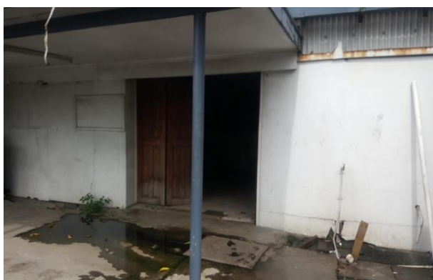
Figure 19.1: Door not secured, leaked sewer line
