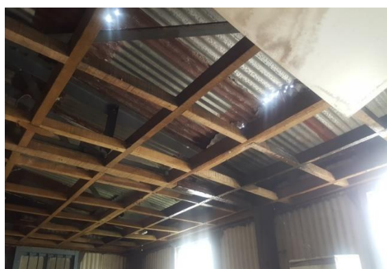
Figure 19.2: Leaked rusted roof without ceiling
