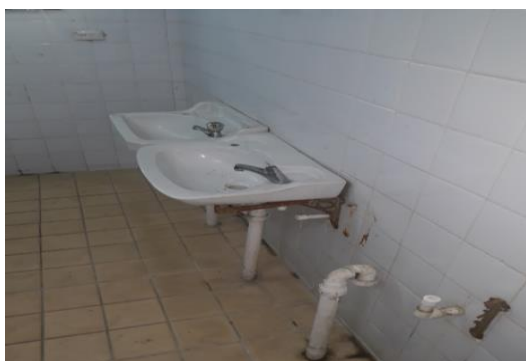
Figure 20.15: Broken taps and wash bowl
