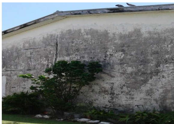
Figure 20.23: Worn out paint
