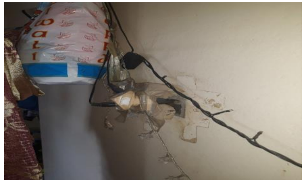
Figure 20.8: Loose power-point
