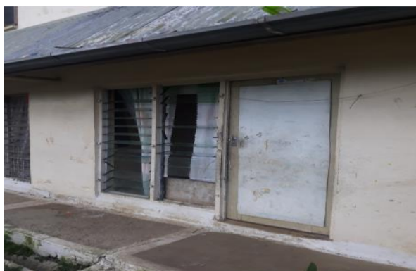
Figure 20.22: Missing louvre blades
