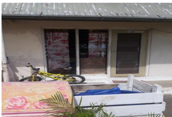
Figure 20.21: Missing louvre blades
