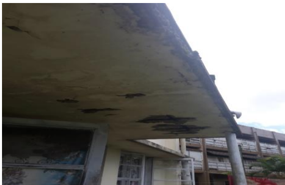
Figure 20.9: Cracks in ceiling
