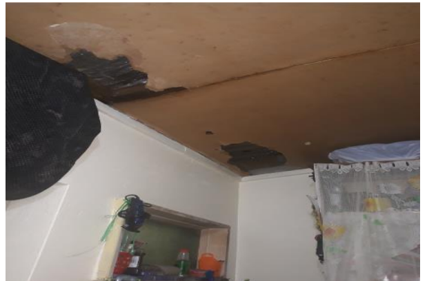
Figure 20.12: Leaking roof
