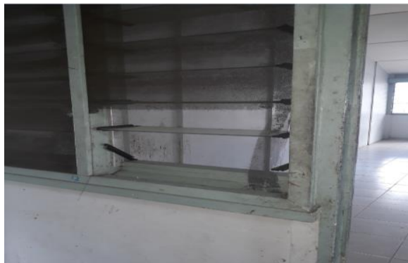
Figure 20.2: Torn mosquito screen missing louvre blades
