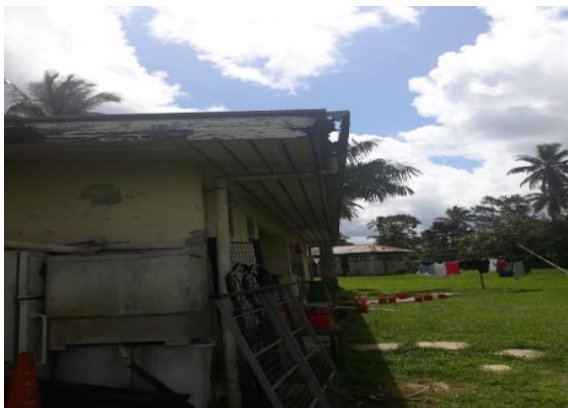
Figure 20.11: Married quarters old guttering
