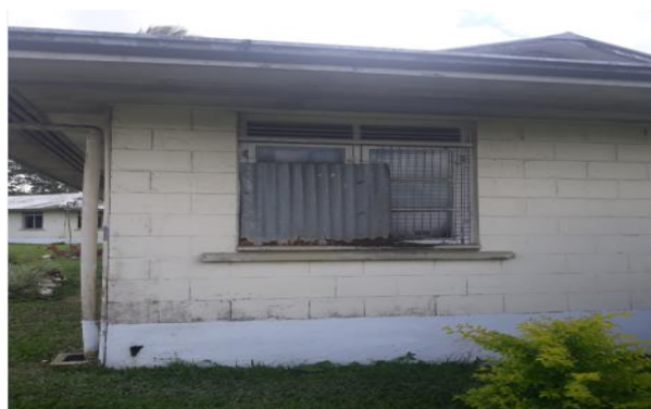
Figure 20.14: Damaged windows for married quarters
