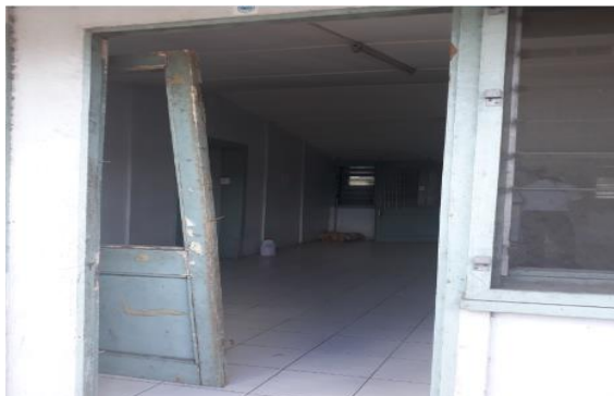
Figure 20.1: Single men quarters door damaged
