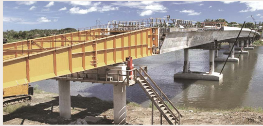
The 40 tonne steel bridge box girder casting mould fabricated by FSHIL, which was used in the construction of the new Rewa bridge completed in 2006.
