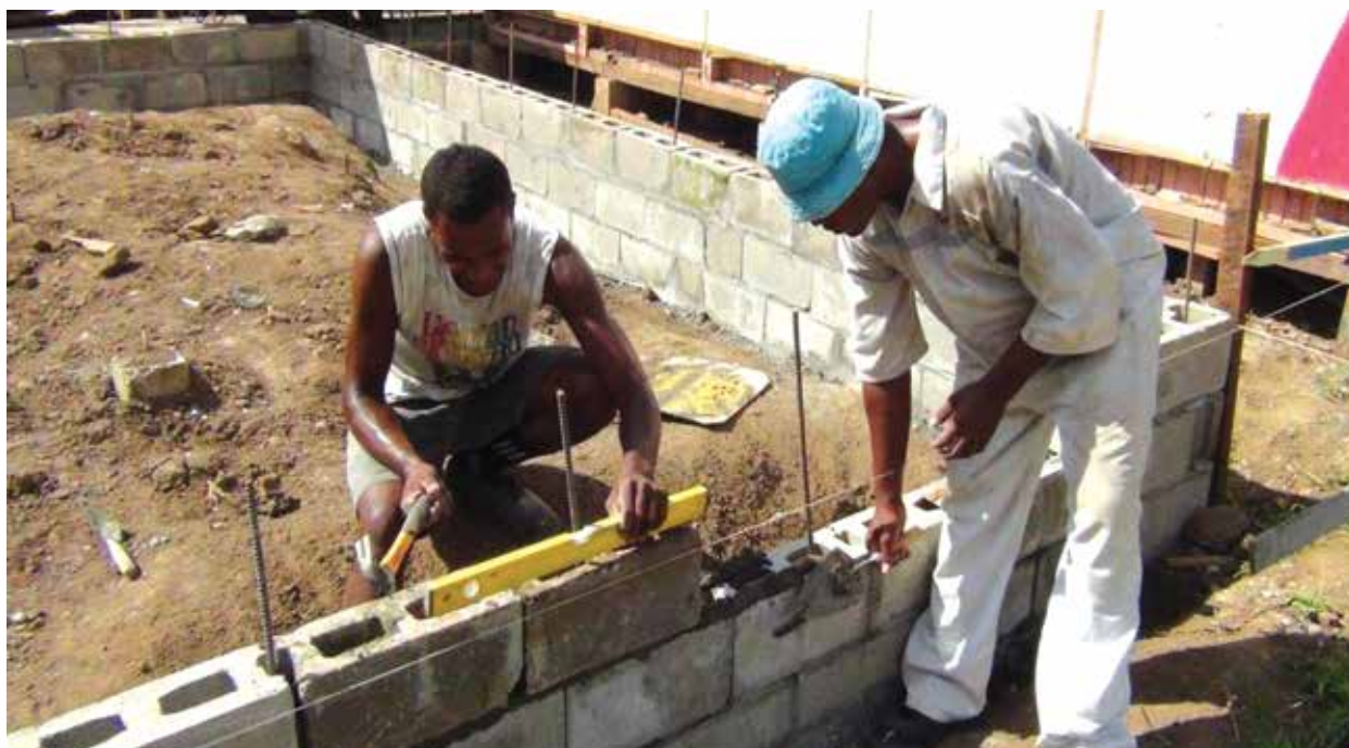
Basic carpentry students of Nasau youth training centre in Sigatoka practicing their acquired trade skill by laying bricks for the new classroom block at the centre
