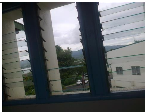
Figure 21.6: Missing louvers at the kitchen walkway
