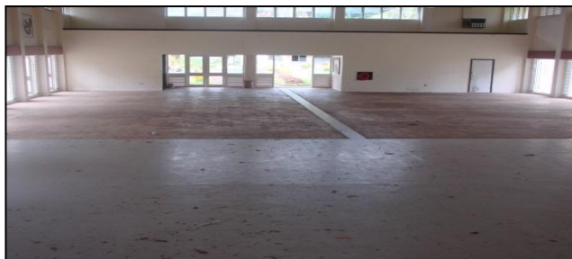
Figure 20.1: Incomplete tiling work in the main hall floor
