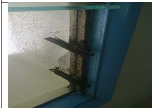
Figure 21.7: Rusty window frame at the kitchen walk way
