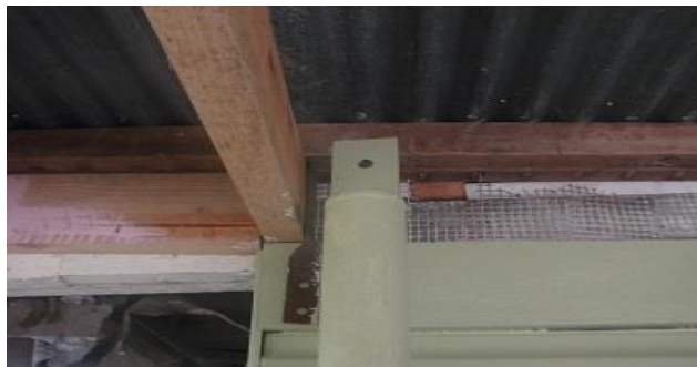
Figure 24.4: Iron post not mounted to the rafter
