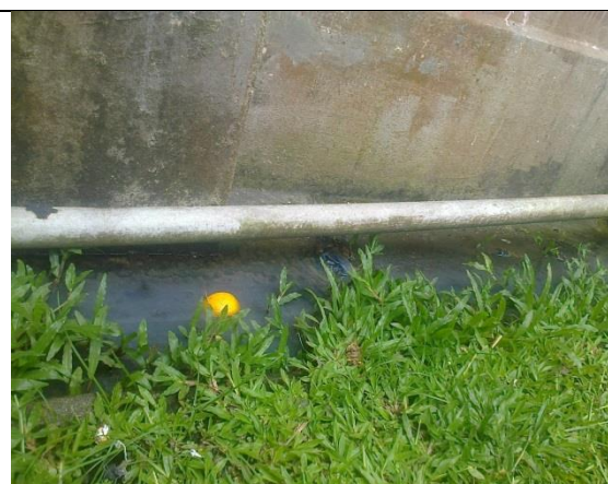
Figure 21.4: Blocked Drains
