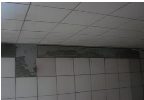
Figure 24.1: Incomplete tiling work
