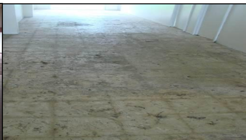
Figure 20.2: Incomplete tiling work hall behind back stage floor
