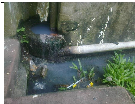
Figure 21.3: Blocked drains due to poor drainage from Kitchen
