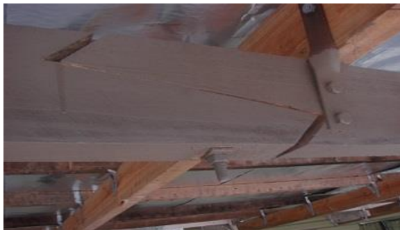
Figure 24.3: The rafter not properly fixed
