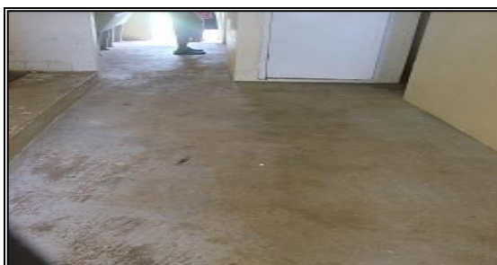
Figure 20.5: Ablution block floor not tiled
