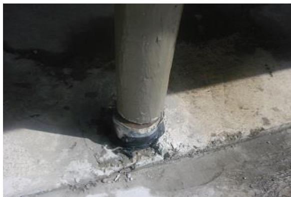
Figure 24.5: Wooden post not properly mounted to the foundation
