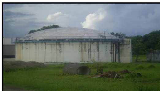
The aluminium dome roof Digester
