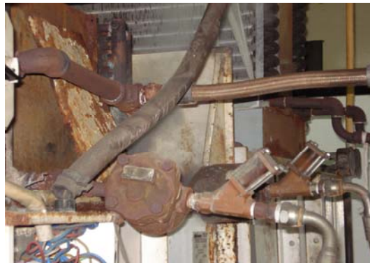
The back of the dryers have started to erode away
