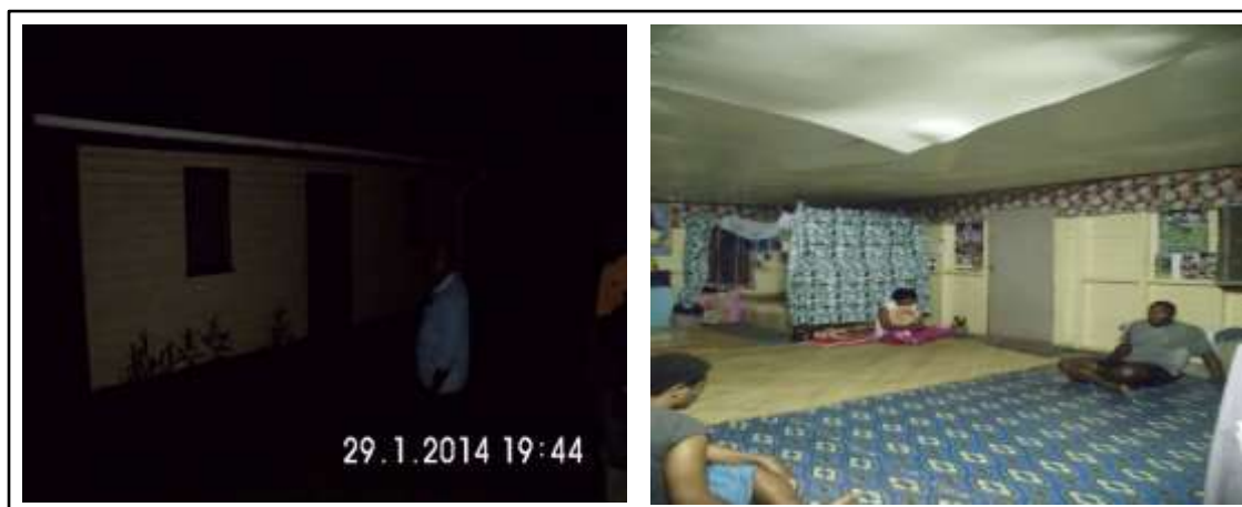
Figure 19.8: Recipient number one (1) – Nagado Village. House is completed and all materials have been received. However, the roof is leaking as shown in the second picture. Due to the leak, one masonite board has started to disengage from the rest of the ceiling.
