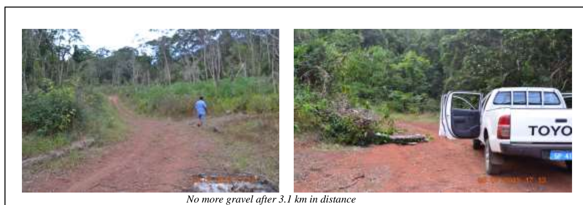
Figure 19.4: Anomalies in Korosomo Farm Road Project
