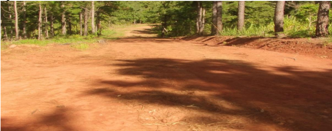
Figure 18.4.2: Naduru Access Road
