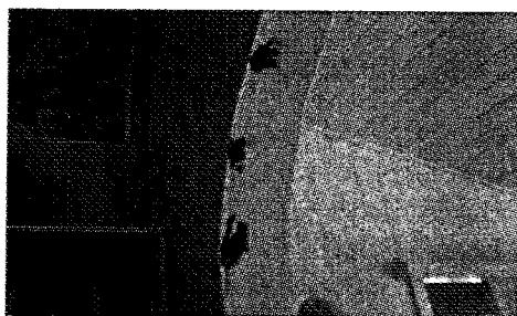
Figure 23.2: Rain water leakage from the Happy Home ceiling
